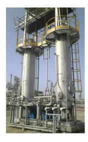
Those units remove  $H_2S$ , VOCs and ammonia from waste air coming from tanks, pits and sumps by a special type of activated carbon.
